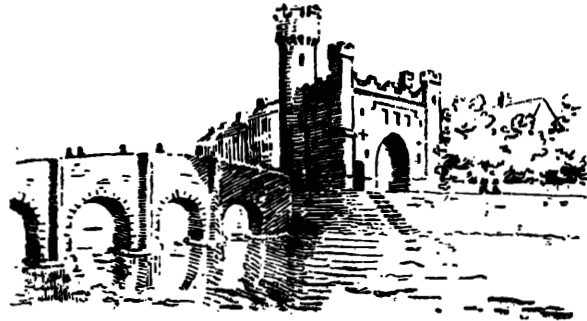
The Last of the Old Dublin Bridges.
